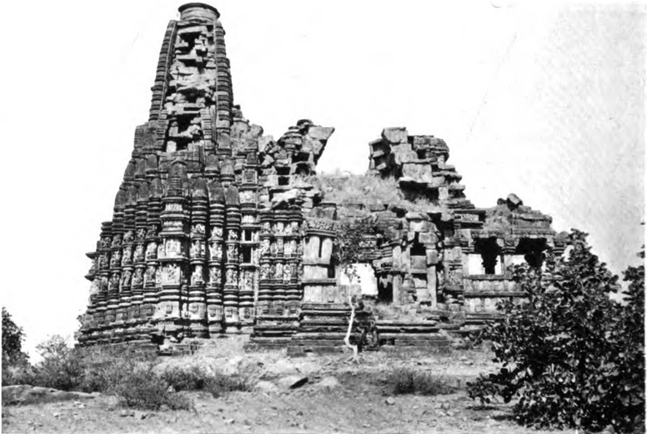
RUIN OF RIVER TEMPLE, NEAR KHAJURAHA. Showing method of construction.
