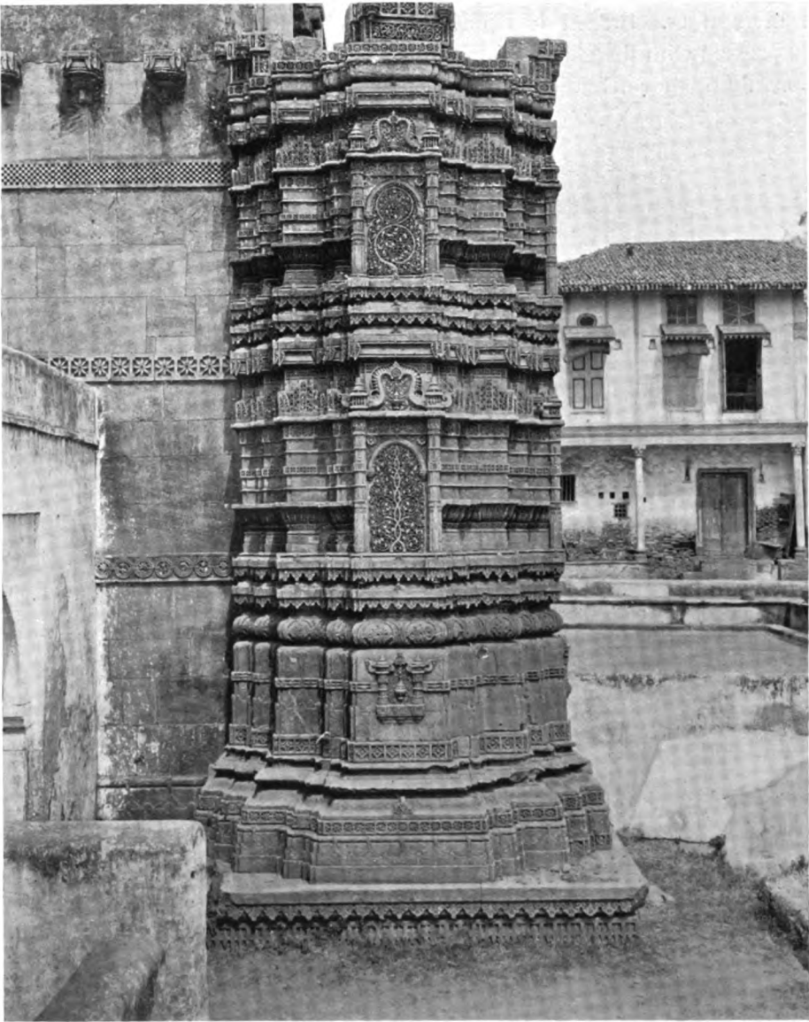
UNFINISHED MISARET SHAIK HASSAN, AHMEDABAD.
