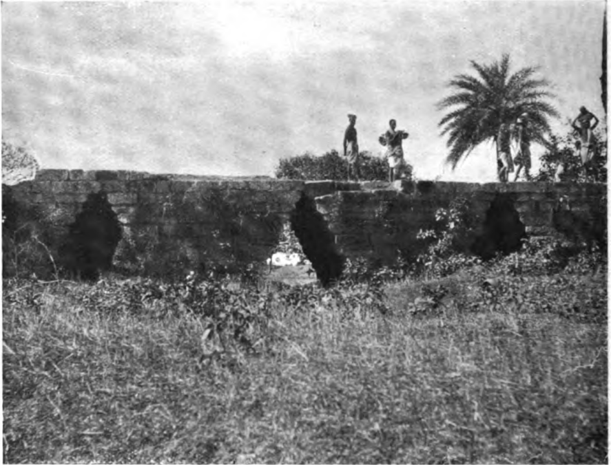
OLD BRIDGE AT JAJPUR.
